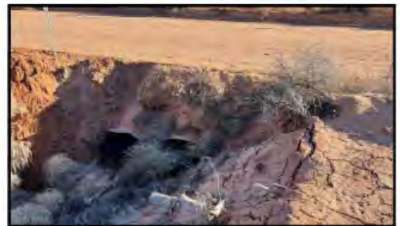
Culvert Cross Drain
