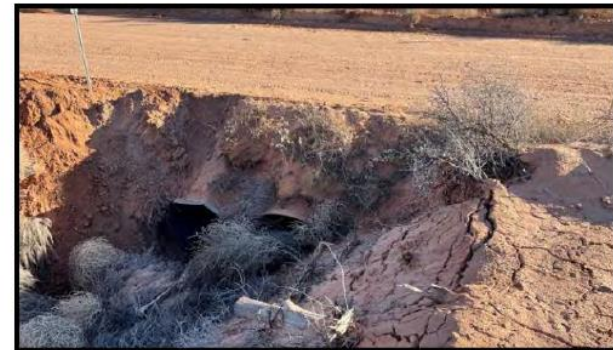
Culvert Cross Drain
