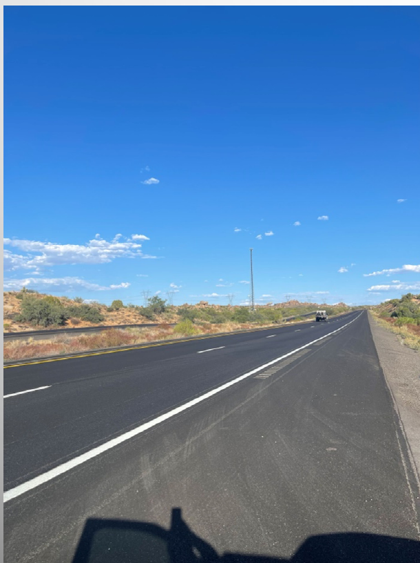
US 93, North of Nothing – South of SR 97
