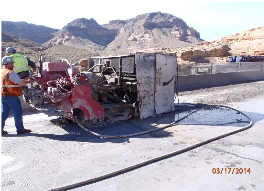
Bridge #7-Hydro-demolition
