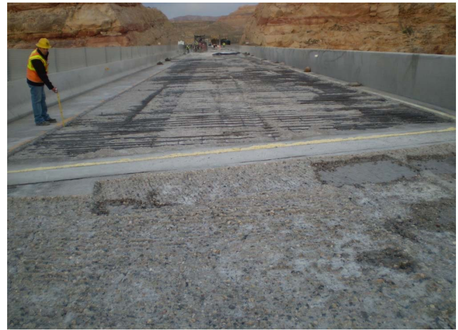
Bridge #7-Hydro-demolition
