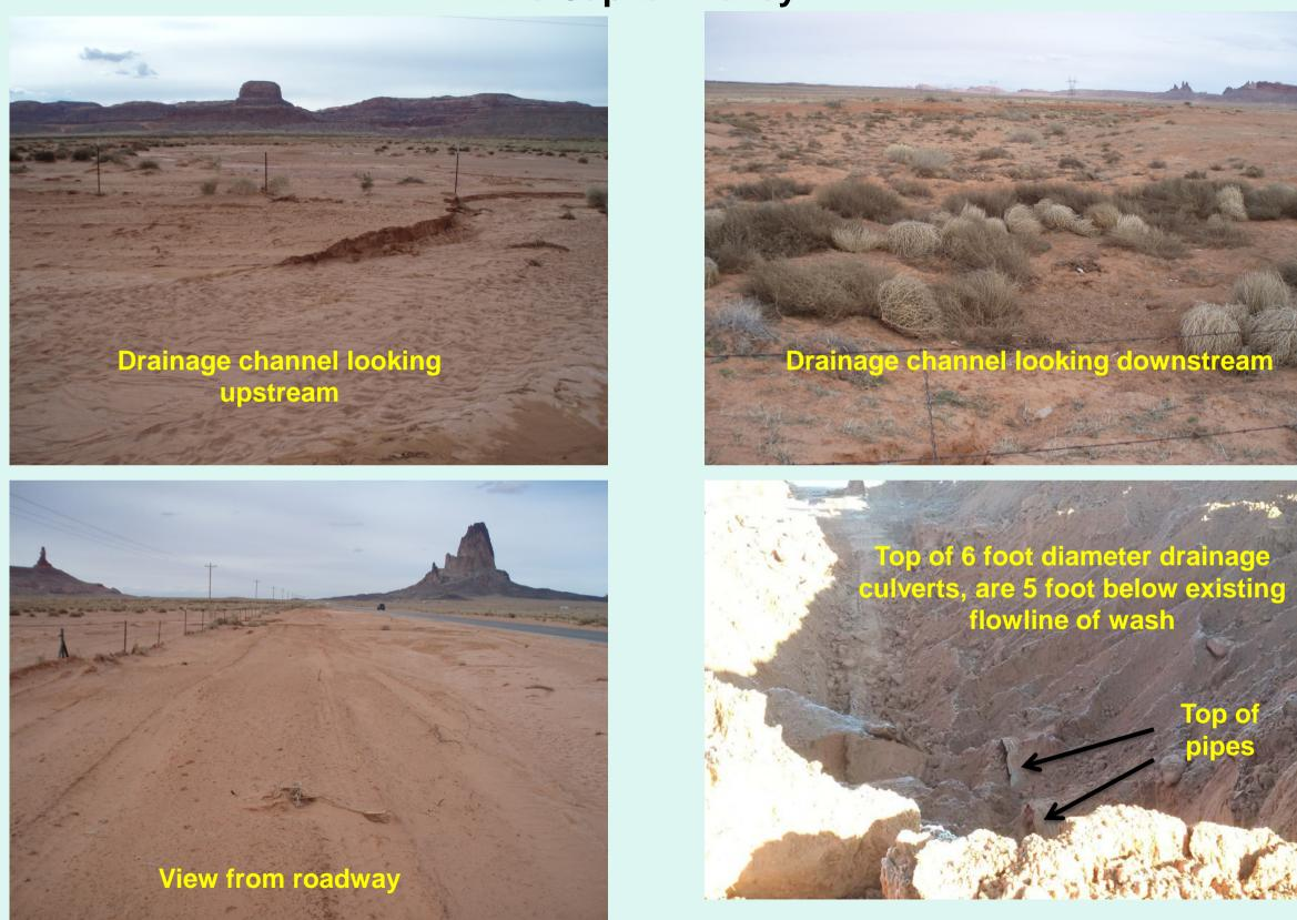
The existing two 72"x74' CMPs that conveyed the wash water under US 163 have been completely silted in and are approximately 5' below the present wash flowline
