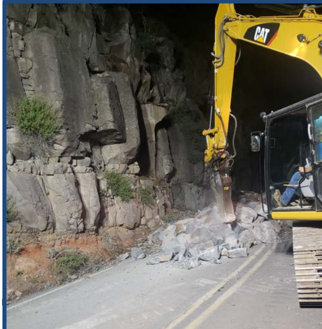
SR89A, Pumphouse Wash Bridge, Rockfall Mitigation, and Erosion Control
