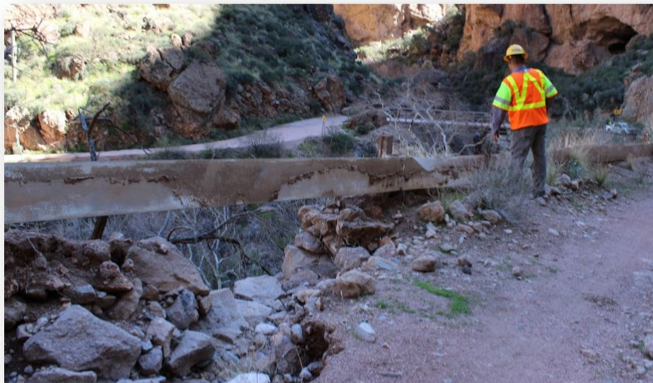
Eroded roadway edges
