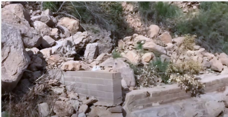
Buried culvert inlets
