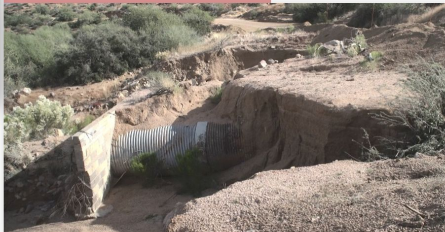
Clogged damaged culverts
