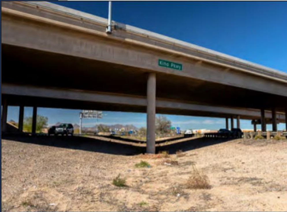
Kino Parkway overpass on I-10 in Tucson
