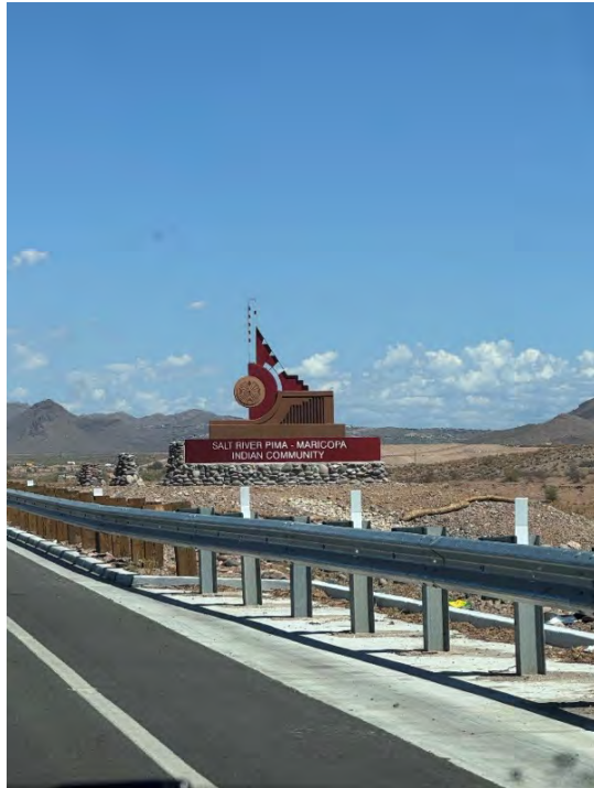
Figure 6: Salt River Bridge
