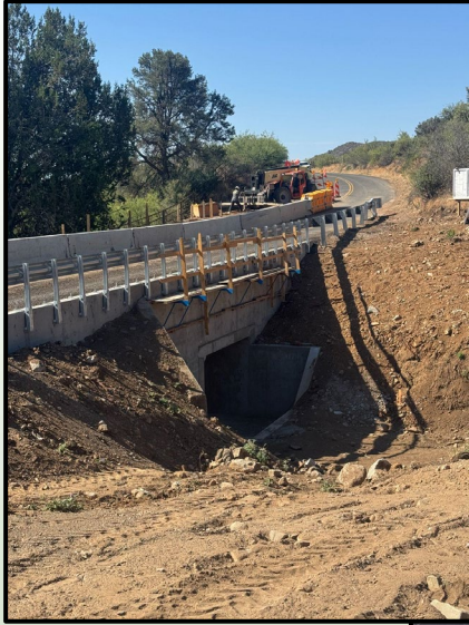
Wash Bridge at Walnut Grove
